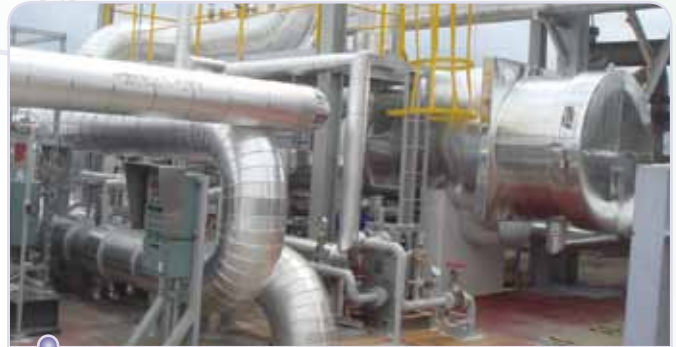
Evaporating Condenser for MVR (Mechanical Vapor Recompression System)
